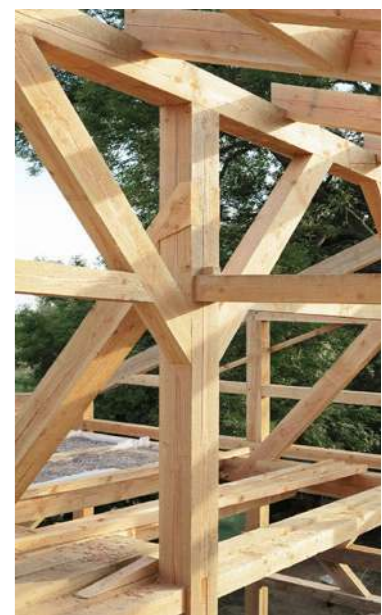
Bauphase – Detail, Foto: © Hans Peter Wieser, Berlin
