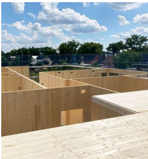
Bauphase, Foto: © Mareike Zabel
